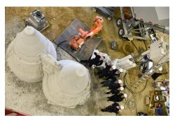
The Penn State Den@Mars shortly after completing the first-ever fully enclosed 3D-printed building structure. IMAGE: NASA
