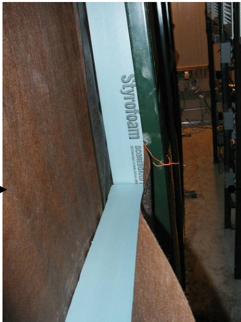
Figure 2-12: Soil insulation / separation
