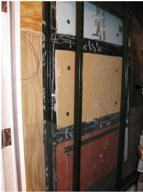
Figure 2-10: Finishing of the exterior
