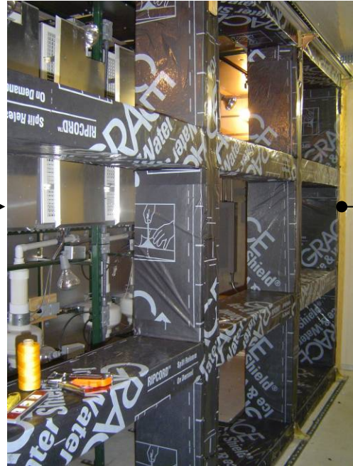
Figure 2-6: Moisture barrier
