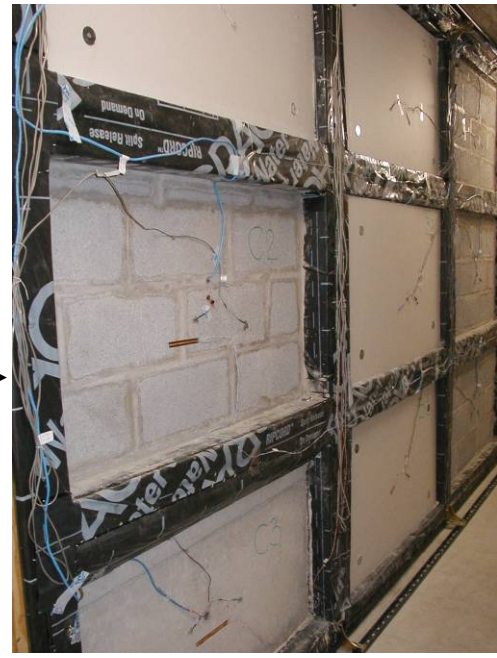
Figure 2-8: Finished test wall
