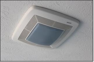
Figure 1: Exhaust only mechanical ventilation.
