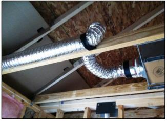
Figure 2: Excessive turns in duct line.
