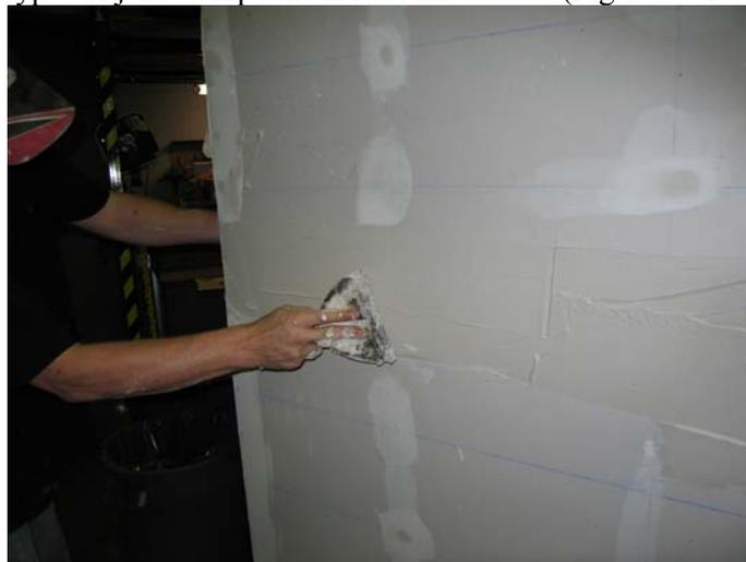
**Fig. 3-18: Professional drywall installer applying joint compound**
