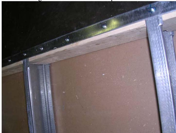
**Figure 3-15: Stiffening of top and bottom steel tracks with wood blocks**
