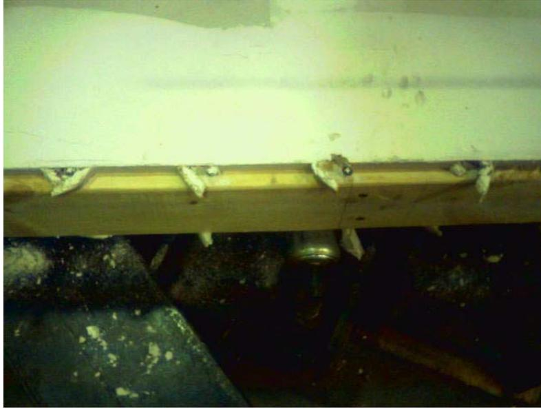
**Fig. 4-38: Drywall screw pullout from GWB**
