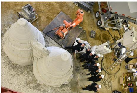
The Penn State Den@Mars shortly after completing the first-ever fully enclosed 3D-printed building structure. IMAGE: NASA
