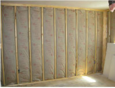
Proper fiberglass batt insulation installation in wall cavities
