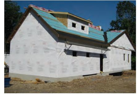
Properly installed housewrap on walls and roof
