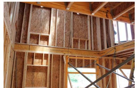
Wood shear wall construction
