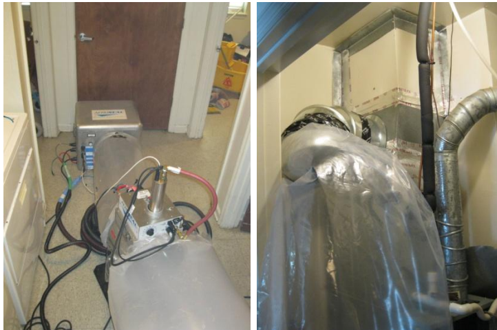
Figure 1. AeroSeal® equipment (left) connected to supply plenum (right).
