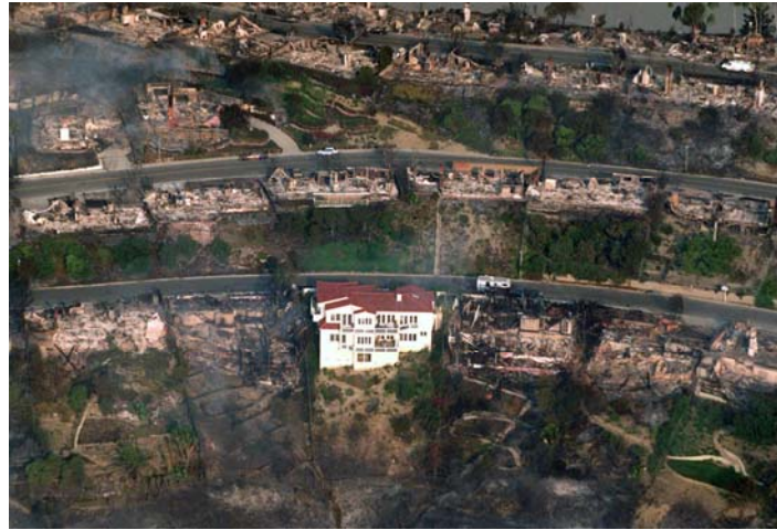
Figure 2. Stucco cladding and eaves along with concrete roof tile helped protect this home during a 1993 wildfire in Laguna Beach, CA (AP Photo/Douglas C. Pizac).
