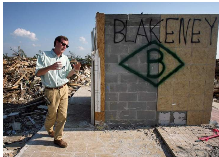
Figure 3. William Blakeney helped build this safe room inside his grandparents' home in Tuscaloosa, AL, before a tornado hit destroying the home and most homes in the neighborhood (The Tuscaloosa News/Michelle Lepianka Carter).
