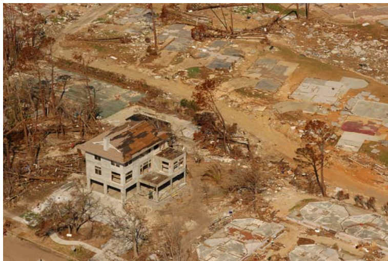
Figure 1. The Sundberg's concrete home survived the devastating effects of high winds and storm surge of Hurricane Katrina (FEMA/John Fleck).
