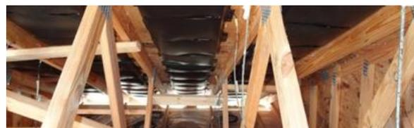
(b) Air Gap Prior to ccSPF Installation
