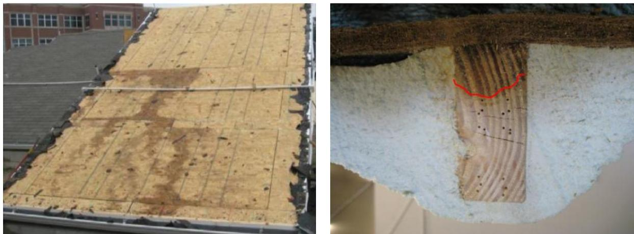
(a) Moisture Buildup in Sheathing (b) Moisture Buildup in Framing Members
