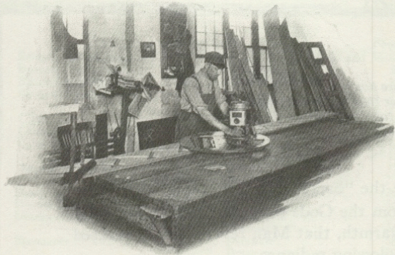
A Better-Built idea—routing (instead of cleating) stair-stringers for fine workmanship, and accurate fit.
