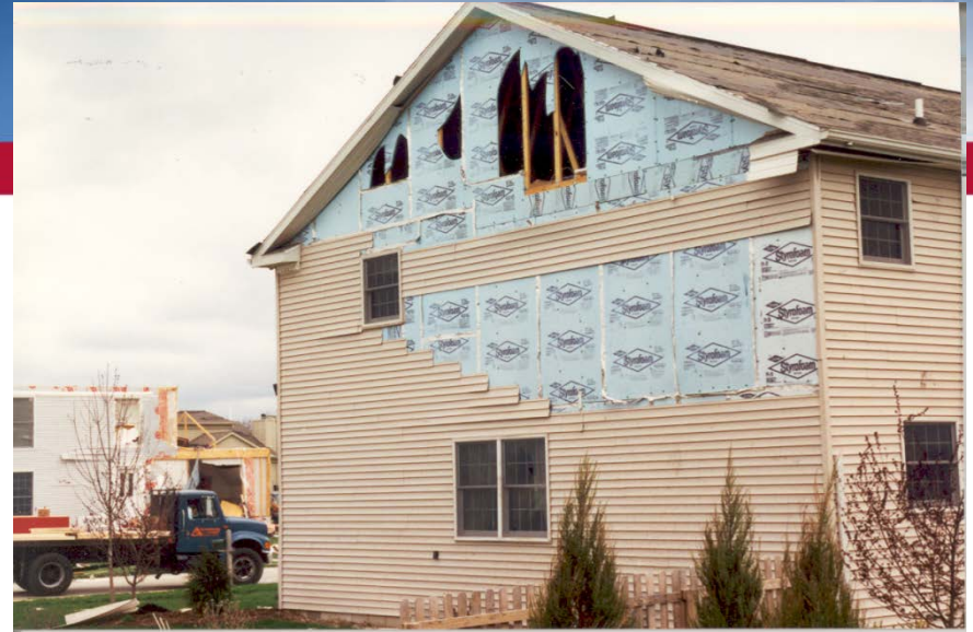
Wind Damage Photos by Rose Grant, AIA, CPCU
