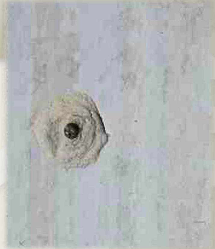
Back of fiber cement board at nail penetration
