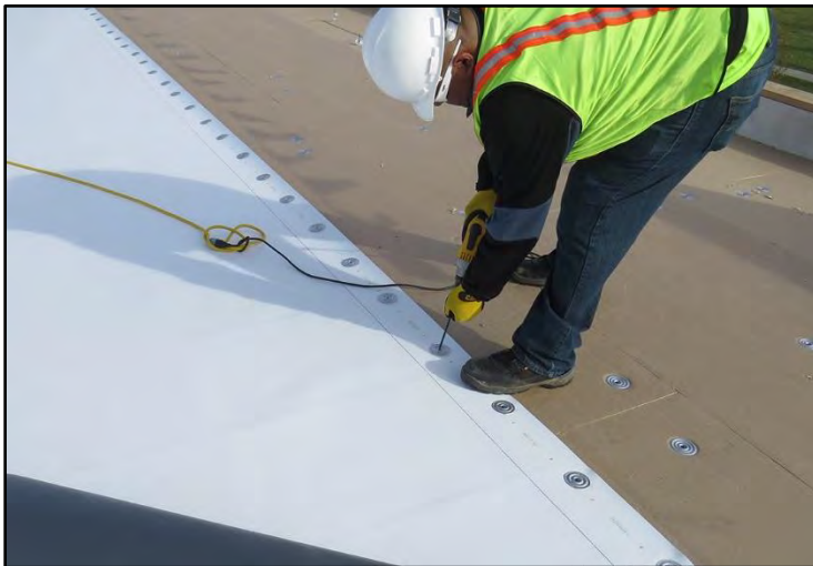
Figure 11. TPO Roofing Assembly (Courtesy of Dykstra, 2016; used with permission)
