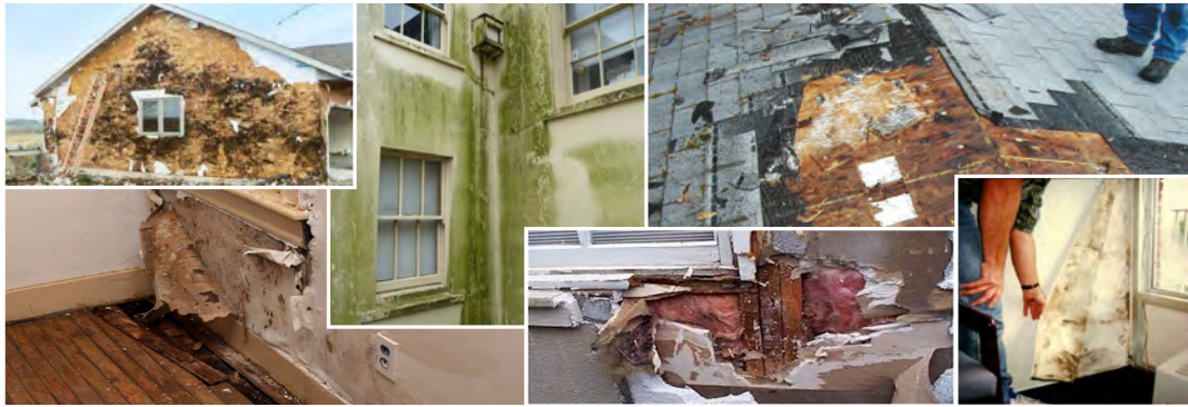
Figure 1. Moisture intrusion in the building envelope (Source: DOE Emerging Technologies Roadmap, 2019).
