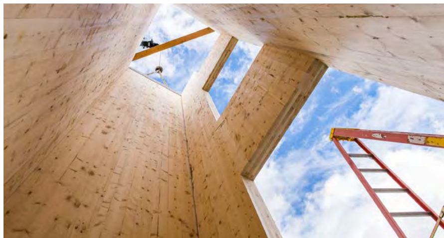
Figure 1. Elevator Shaft Constructed by Smartlam (Photo Credit: Smartlam)
