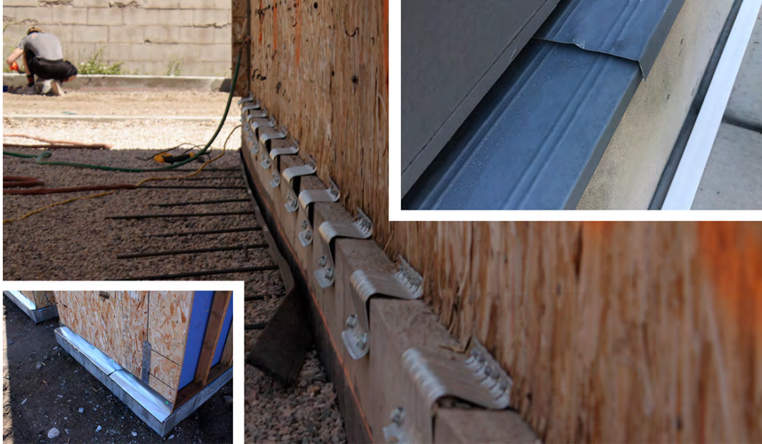
Figure 6: Building officials requested additional brackets as a result of ignoring required building inspections, leading to a flashing detail that directs water behind the façade. Note the considerable concrete ledge at the bottom of the SIPs, where the concrete was supposed to be flush with the exterior OSB above, which would have also allowed using simple seismic strips instead of the heavy brackets.
