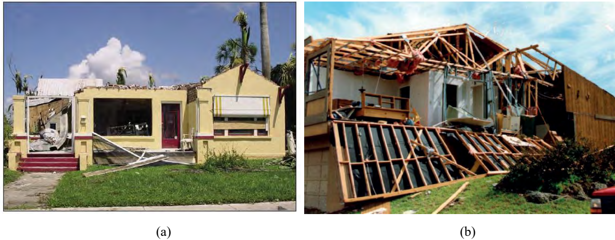
Figure 1. Wind-induced damage to structural members (FEMA P-488): (a) severe structural damage due to pressurization during Hurricane Charley, 2004; (b) severe damage to roof, structure, and gable end wall during Hurricane Andrew, 1992.
