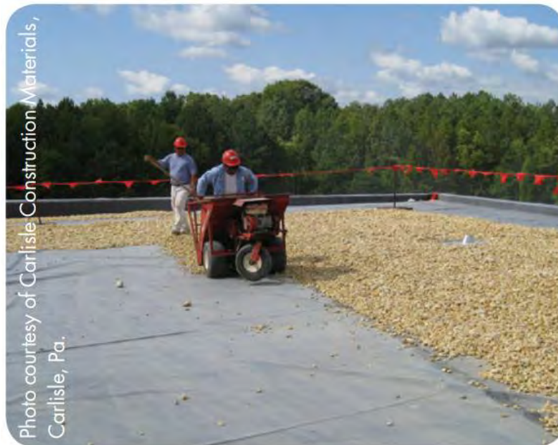
Figure 7. Ballasted EPDM Roofing Installation (Courtesy of Goodman, 2013; used with permission)
