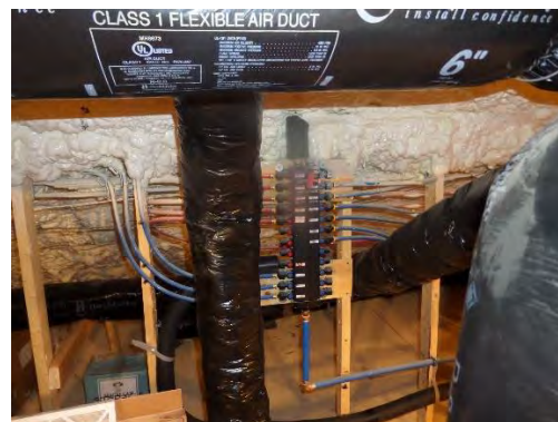
Figure 10: Manifold that routes on-demand hot and cold water to the various plumbing fixtures in the house.
