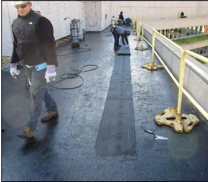
Figure 5. Mod-Bit Installation
