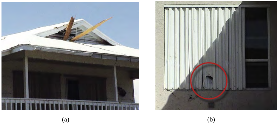
Figure 5. Damage due to windborne debris to building envelopes during Hurricane Charley, 2004 (FEMA P-488): (a) impact of structural wood members in the gable end, Pine Island; (b) a roof tile punctured the shutter, Punta Gorda.
