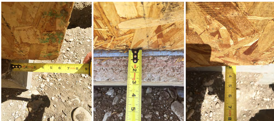
Figure 5: SIPs sit considerably off of stem walls due to inaccurate concrete formwork and concrete pour.
