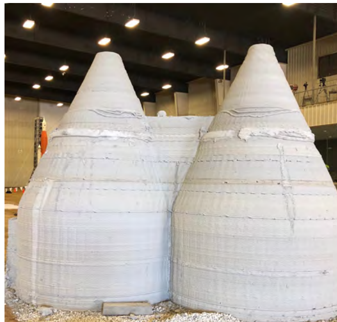
Figure 11: Final 3D printed concrete structure at the actual construction level.
