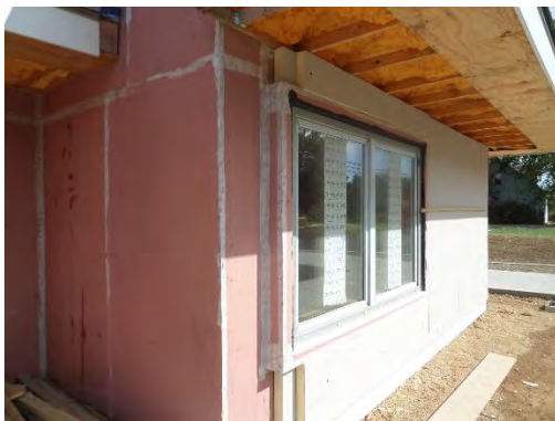
Figure 9: Window “box” partially exposed as continuous insulation is installed. Note tape at all sheathing joints and around window. Tape and sealant were installed by first timers.
