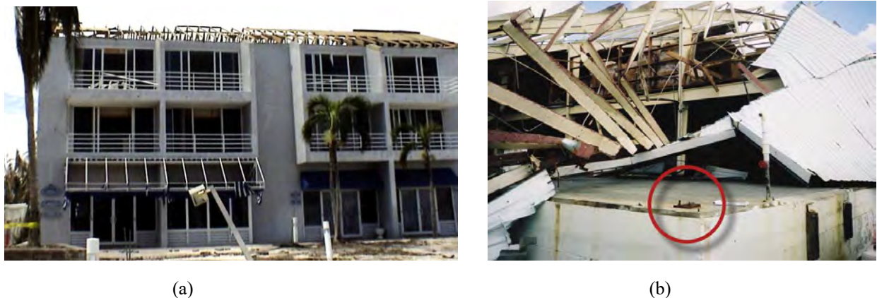
Figure 10. Wind-induced damage to concrete and steel frame buildings during Hurricane Charley, 2004 (FEMA P-488): (a) damage to a multi-family building roof deck with inadequately supported and braced overhang; (b) roof framing failure and gable end wall collapse due to insufficient lateral supports.
