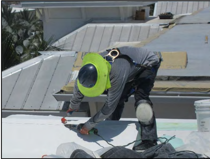
Figure 9. Hand Gun Welding
