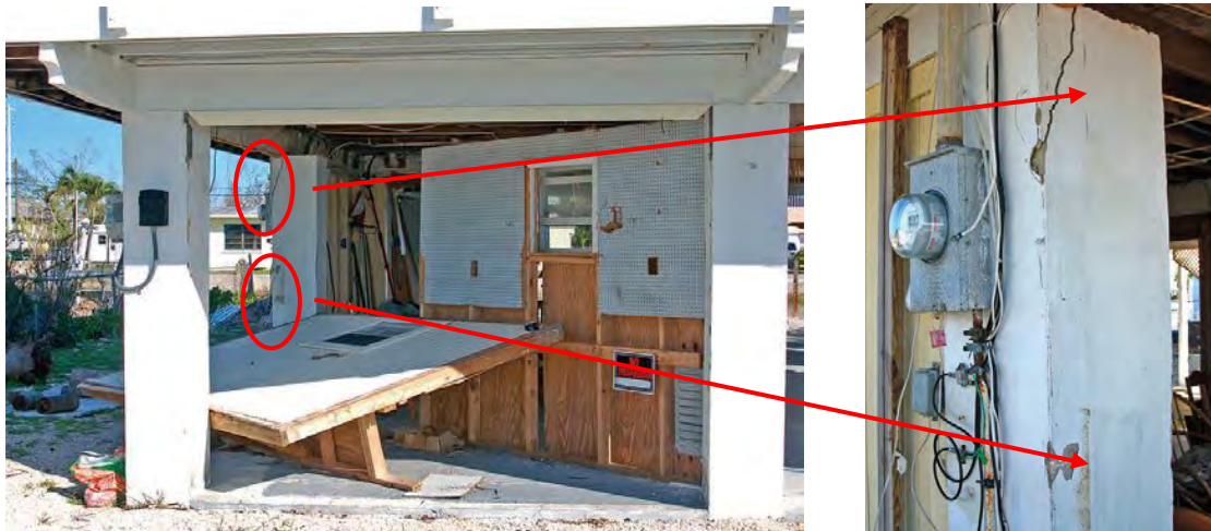
Figure 7. Severe damage to columns due to inappropriate connections between the breakaway wall and main structural members during Hurricane Irma, 2017 (FEMA P-2023).
