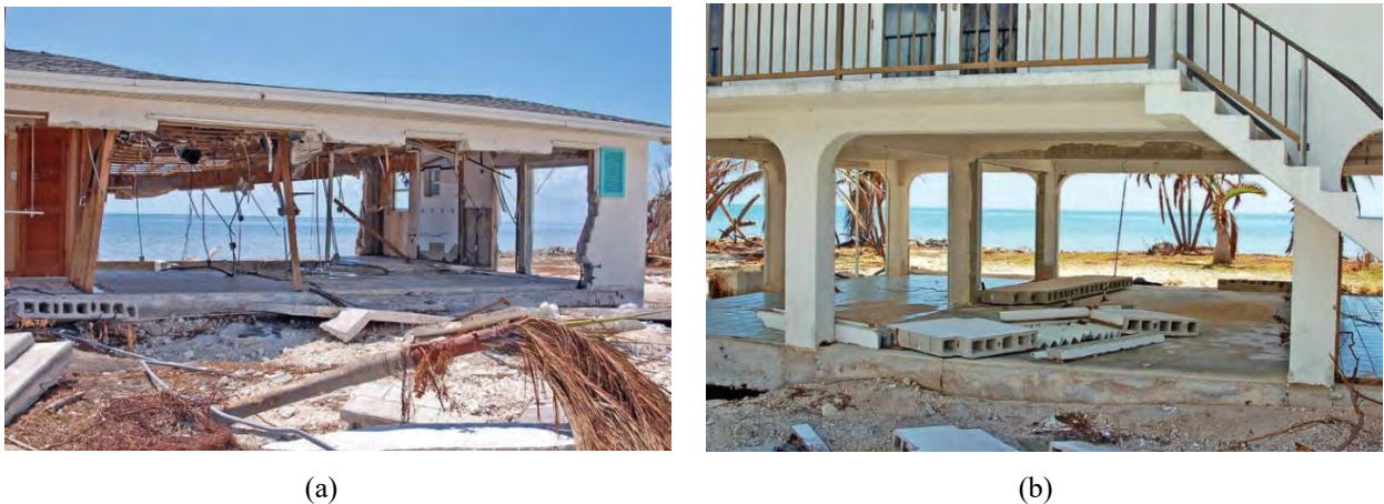
Figure 6. Performance of breakaway walls for houses located in Big Pine Key, FL during Hurricane Irma, 2017 (FEMA P-2023): (a) severe damage to masonry walls of a slab-on-grade house due to lack of breakaway walls; (b) limited damage to the house due to the role of breakaway walls during the flood event.
