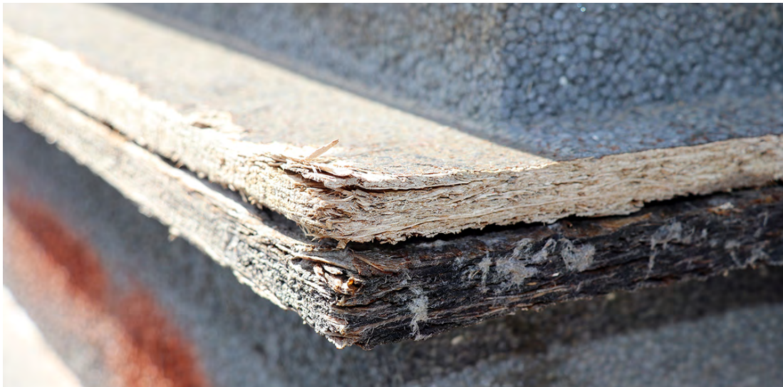
Figure 3: Deteriorated SIPs due to prolonged weather exposure.
