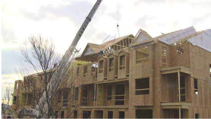
Figure 4. Truss Rafting of Roof Section Onto Townhouse
