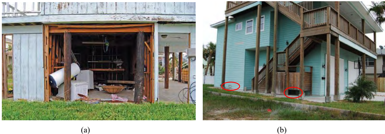
Figure 8. Performance of elevated houses with enclosure with/without openings during Hurricane Harvey, 2017 (FEMA P2022): (a) extensive damage to the enclosure due to lack of flood openings; (b) elevated house suffered minor damage due to having flood openings for enclosures below the BFE.
