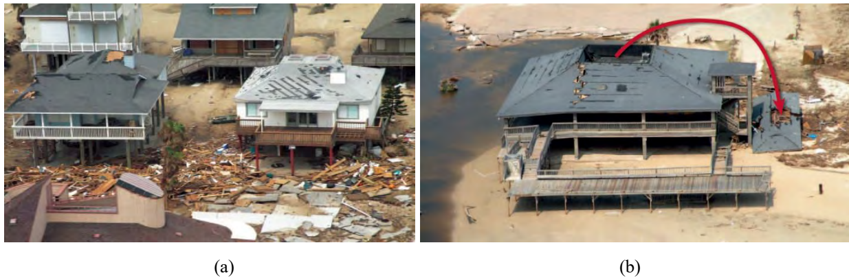
Figure 4. Wind-induced damage to the roof structure of elevated houses during Hurricane Ike, 2008 (FEMA P-55a): (a) roof covering and sheathing damage at roof edge and roof corners (Galveston, TX); (b) total collapse of the roof structure (Galveston, TX).
