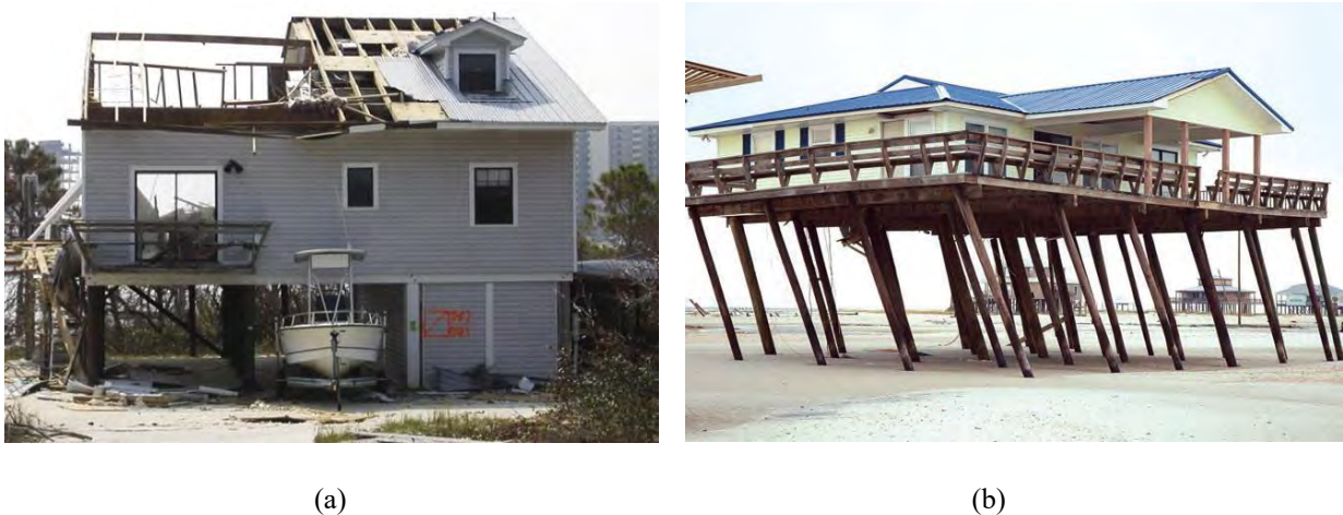
Figure 4. Structural damage to elevated houses due to the wind during Hurricane Katrina, 2005 (FEMA 549): (a) severe damage to the roof framings and gable end wall; (b) excessive lateral displacement due to the insufficient pile embedment.
