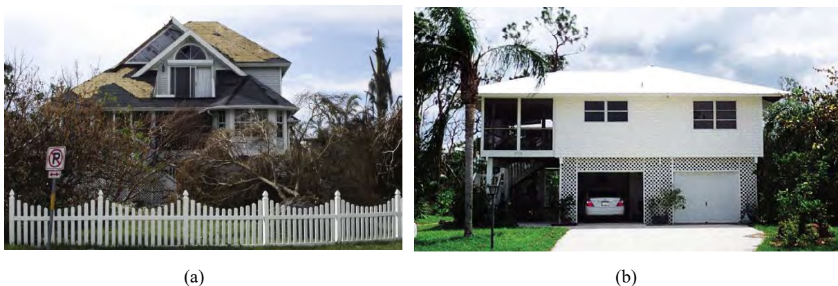
Figure 2. Typical roof covering loss during Hurricane Charley, 2004 (FEMA P-488): (a) asphalt shingle roof covering loss (Captiva Island); (b) undamaged metal panel roof (Pine Island).
