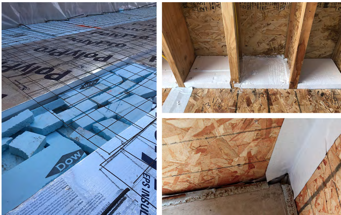
Figure 8: Compromised insulation and air tightness measures. Left: non code-compliant usage of left-over XPS pieces; upper right: hand-cut EPS used to fill the rim board cavities instead of using closed-cell Icynene; lower right: improper tape used on the inside of the SIPs to achieve better air tightness.
