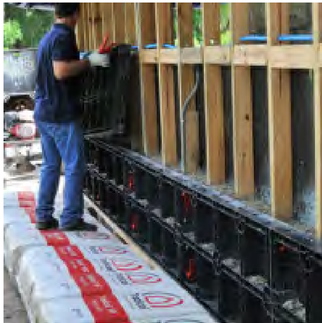
Figure 4 Formwork for placement of cast in place hempcrete to confine studs (Courtesy of American Lime Technology http://www.americanlimetechnology.com/clayton-house/ )
