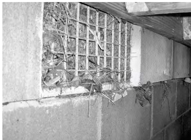
Figure 9. Typical flood opening clogged by flood-born debris (FEMA 2008).
