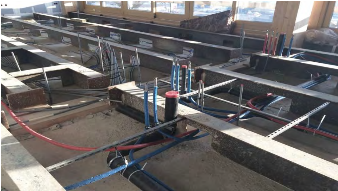
Figure 5: Hollow Slimline floor system with free positioning of drains and wiring. ( https://www.slimlinebuildings.com/PDF/en/news/building-for-eternity.pdf )
