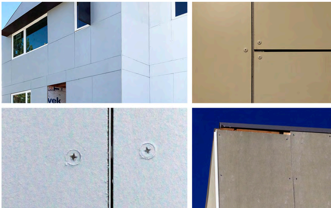
Figure 9: Façade construction as originally designed (upper right image of a mock-up) and as executed by SLVHFH. Lower right image: note the missing flashing at the rooftop, with wood directly exposed to the weather, as it appears in many other locations on the façade.
