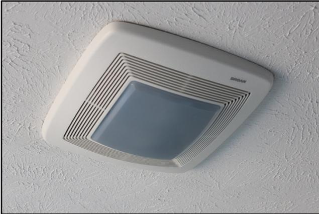
Figure 1: Exhaust only mechanical ventilation.
