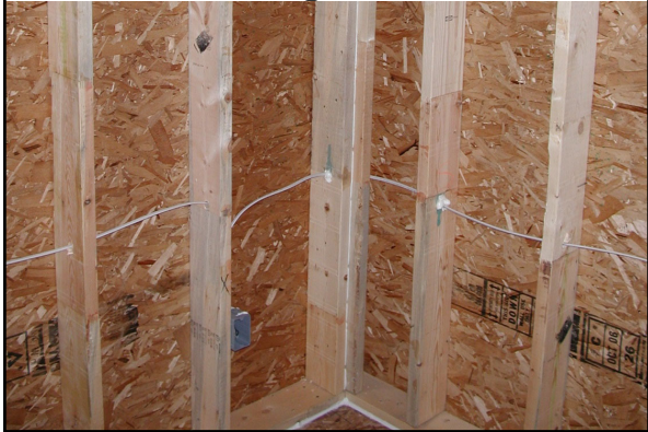
Air sealing at corners
