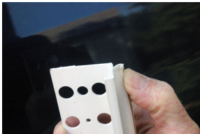
Casing With Expansion Flange Ready to Caulk
