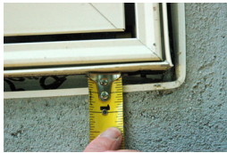
Casing Bead Installed
