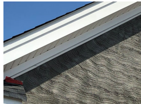
Installed To Trim Under Soffit
