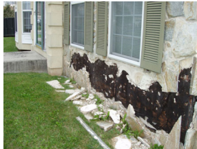
Moisture Failures Appear First in Hygroscopic Claddings
