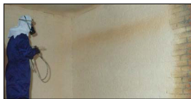
Spraying over an interior masonry wall
