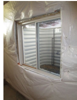
Don't drain access window into basement gravel or sump
