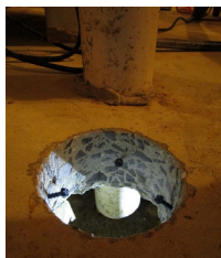
Radon vent pipe jammed in the dirt
