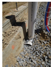
Radon Pipe installed below the gravel
